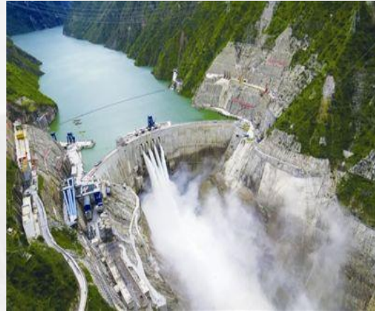
Cambodia Tatai Hydroelectric Power Station
